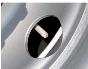
Broken plastic valve extension
