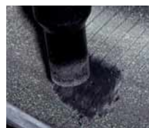
4. Remove any sanding dust with a vacuum cleaner.
