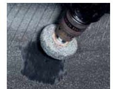
3. Sand without applying pressure (remove any ridges). Maximum speed: 5000 rpm.
