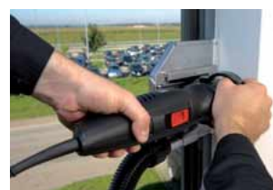
The joint cutter can be guided diagonally while cutting so that the cut line is directly above the old window frame. Otherwise, the distance from the old window frame is 7 - 8 mm. Ideal for the frames of today's insulated glass windows.
